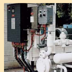
Top left: Cogeneration for Victorian hospitals Centre: Final commissioning, Varanus Island Bottom: Stand alone flash gas compressor, Varanus Island
